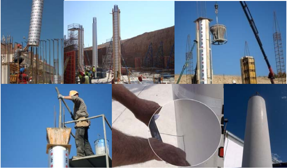
Picture 2. Laying in site of TBT formworks.
